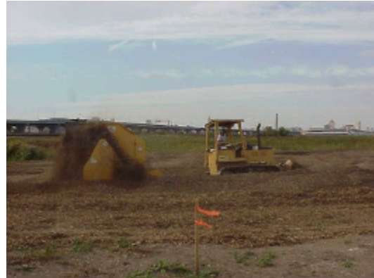
Land biotreatment operation at Milwaukee Harbor
