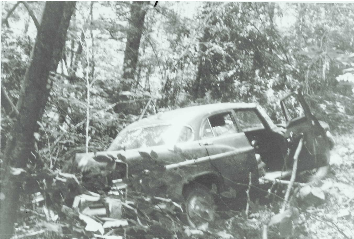
Site of '56 Chrysler loss – There it lay!
