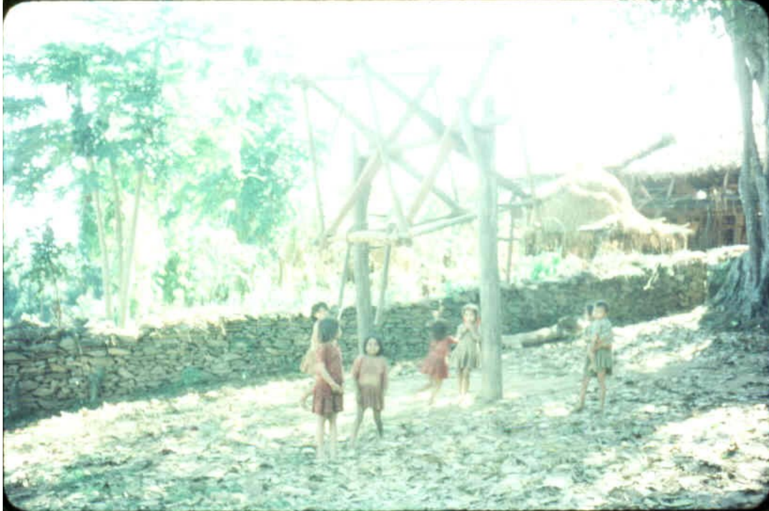
Possible spindle for braiding cable for bridges (?)
